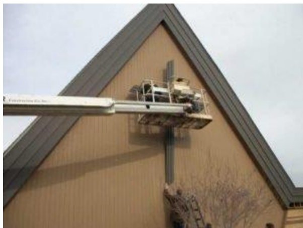
LCMS cross is lifted into position in 2012.
